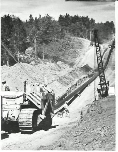
New Alberta pipeline completed in 1961 connects Kaybob oil field with Edmonton by 161-mile, 12-inch pipe. A layer of coal tar enamel reinforced with fibreglass protects the pipeline when buried.
